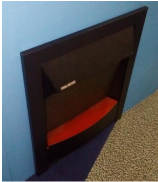
Option 1. Fully recessed installation
